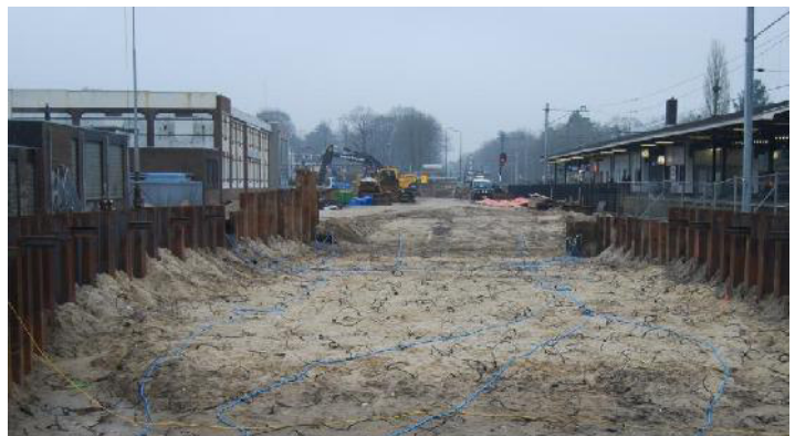
Soil grouting with silicate hardener mixture
